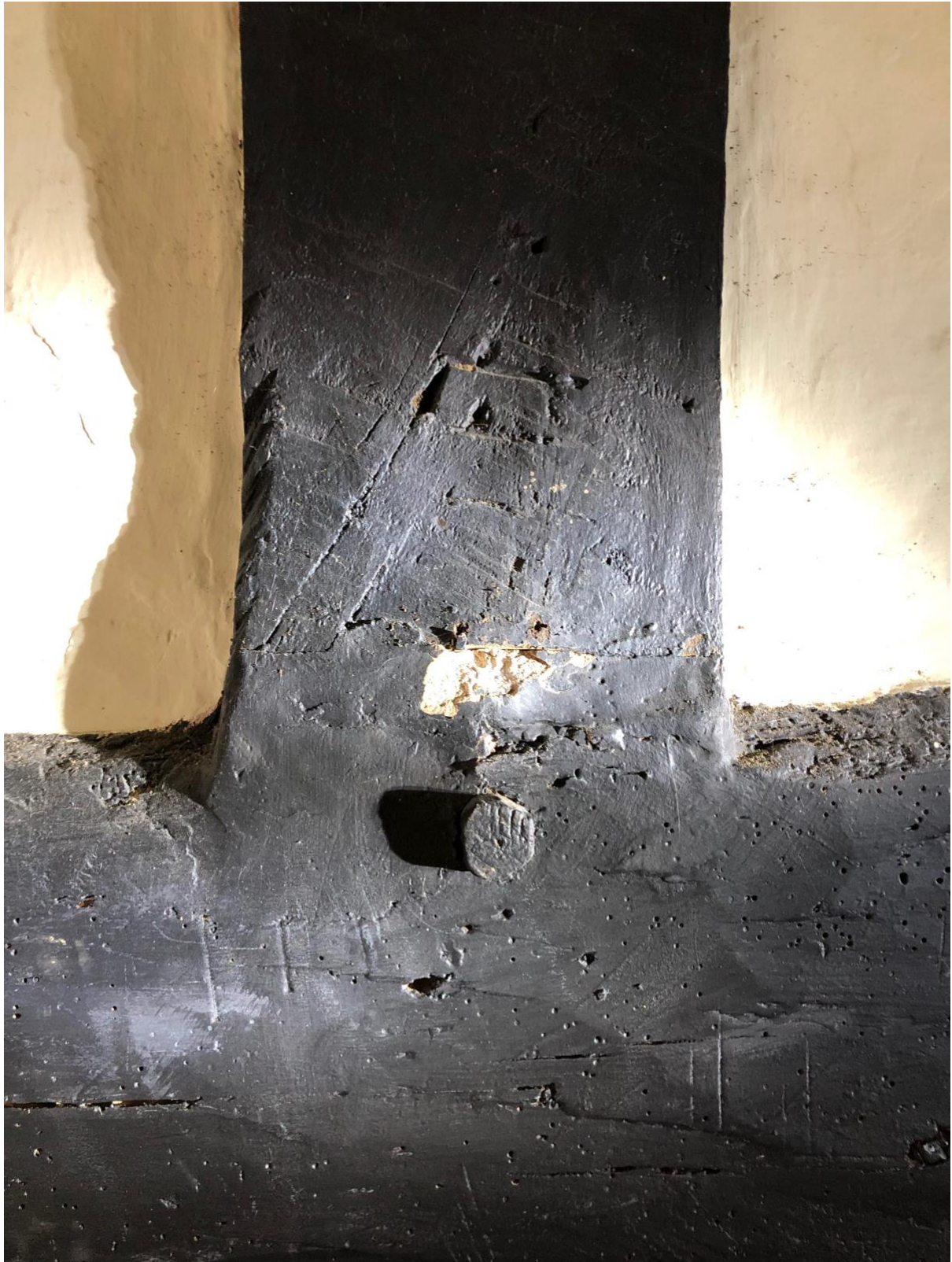
Figure 13, Carpenters assembly marks, in this case II.
