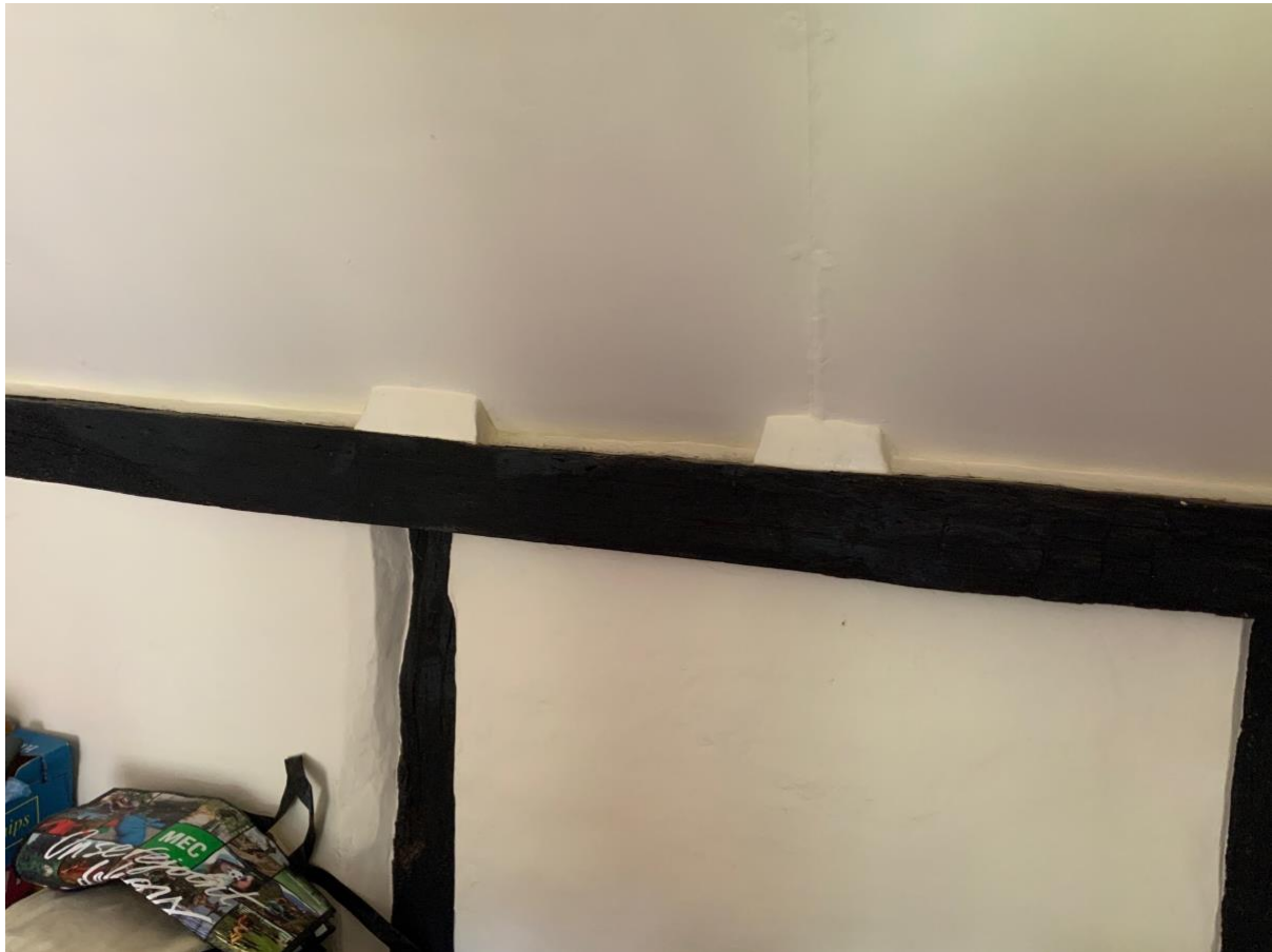
Figure 7, unusual plaster lumps.
