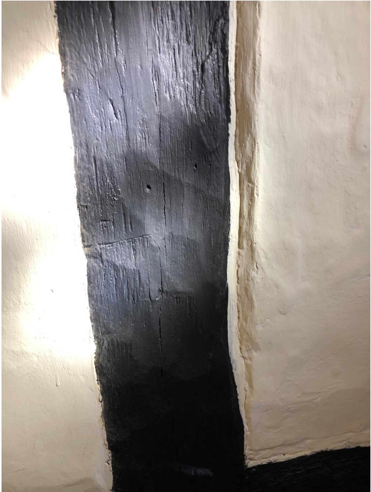
Figure 12, this timber shows evidence of the use of a 'Adze' a shipwrights tool.
