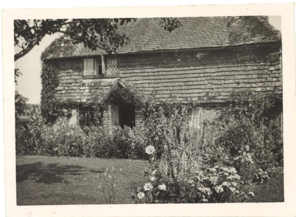
Figure 18, South Elevation of both main range and West wing from 1937.
