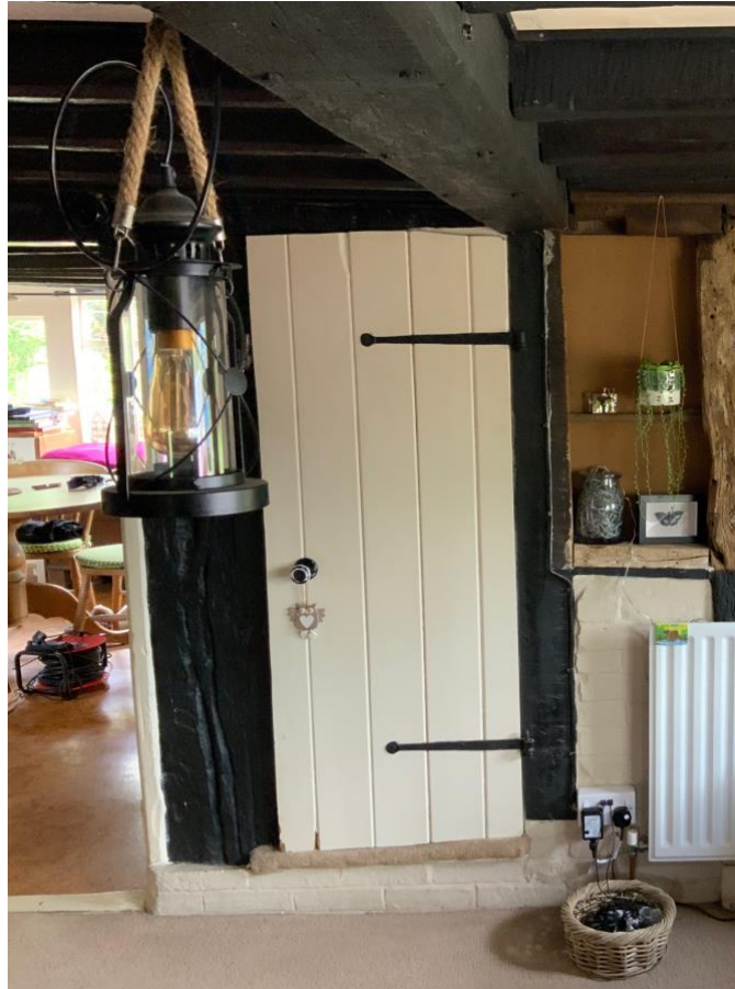
Figure 16, Door to base of stairs from Lounge. (author 2019).
