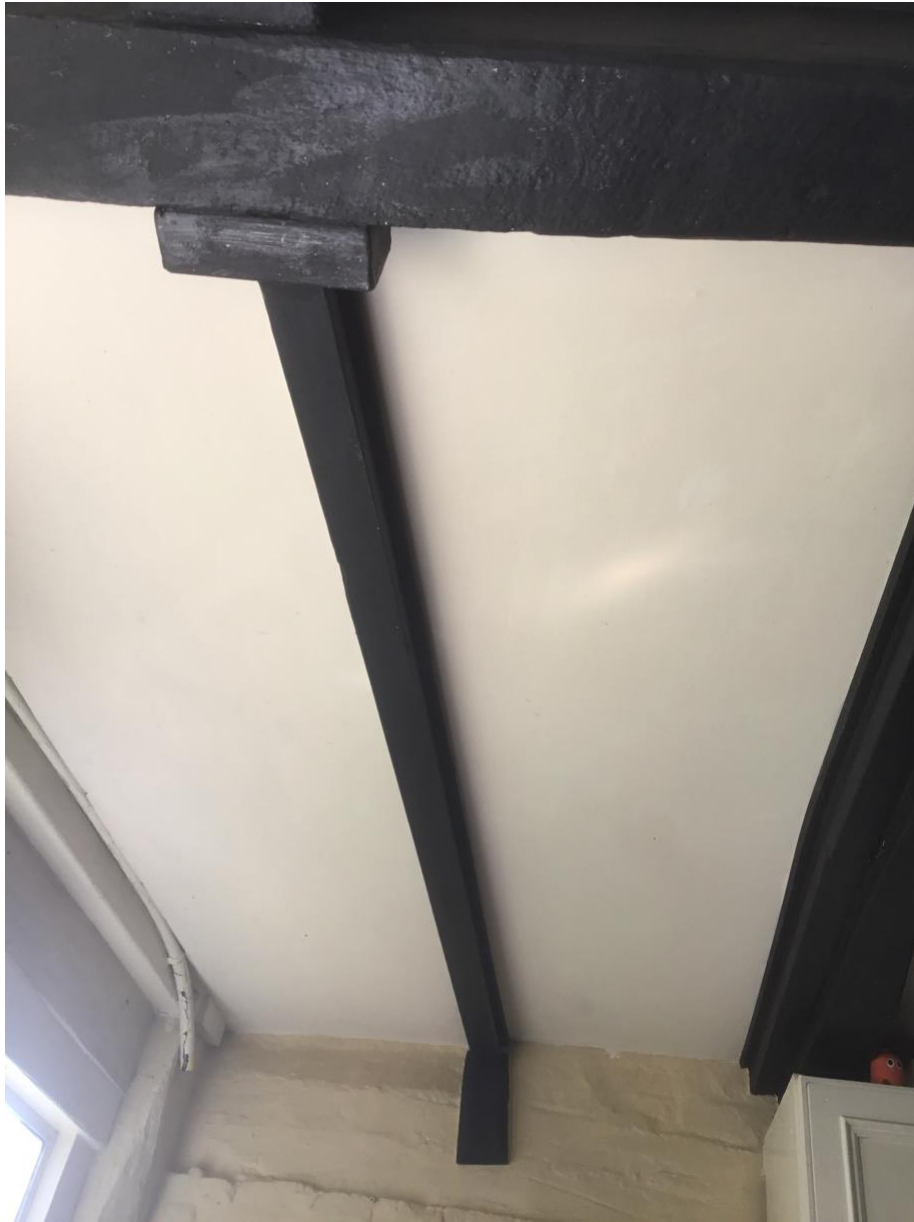
Figure 24, Removable Joist found in South East corner of Bay I (Deborah Woollin 2019).
