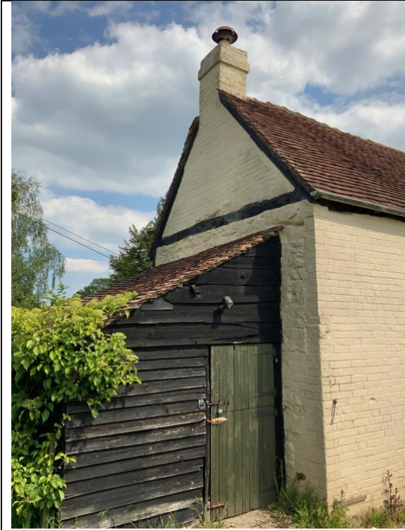
Figure 20, North gable end. (Author 2019)
